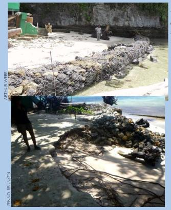
Unfortunately, the site that was chosen for the composting toilet was in the highly active zone that has shifted around regularly. While it appeared there was an "erosion" problem, the sand was merely moving through its natural process to a different location just south of the structure, based on shifting wind conditions. While the movement of sediment was threatening the structure itself, the sediment had not been lost.
