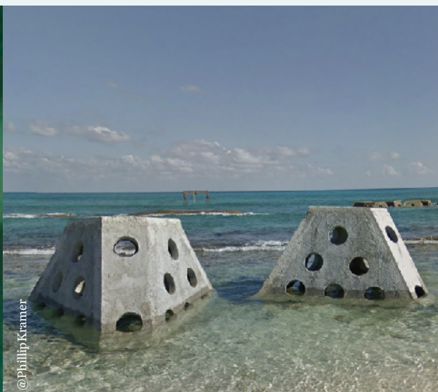
FIGURE 9 | WADs used in the construction of a submerged breakwater located in the Mexican Caribbean, specifically in Puerto Morelos, outside the protected area (Silva et al. 2016).
